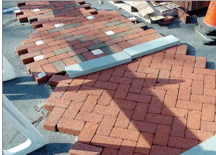
Christopher South/Cape May Star and Wave Top, the 300 block of the Washington Street Mall is being prepared for concrete. Bricks shown above will be placed on top of the concrete to form the new walkway and sidewalks.
