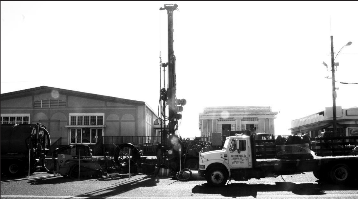
A contractor bores a test well to find the level of geothermal energy that can be garnered for the new Convention Hall.
