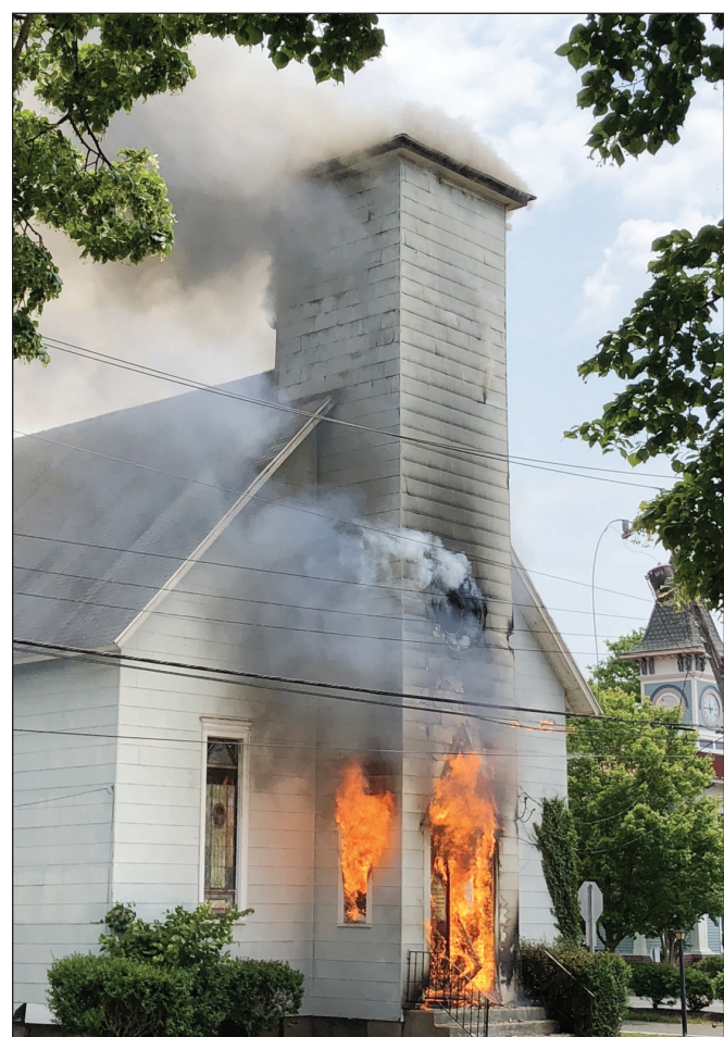
Jack Fichter (file)/CAPE MAY STAR AND WAVE The bell tower at Allen AME Church in Cape May was destroyed by fire in June 2018. The city purchased the structure, conducted some restoration and leased it to a theater company.
