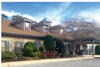
Cape May Court House 106 Court House South Dennis Road
