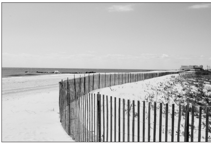
Cain Chamberlin/Cape May Star and Wave Above, snow fence helps maintain the dune structure as part of Cape May's beach protection efforts. Congressman Frank LoBiondo has to fight for federal dollars every year for beach replenishment efforts.
