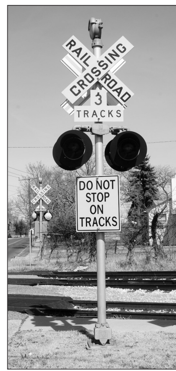
Railroad crossing warning signals, including the crossbuck device at the top of the pole
