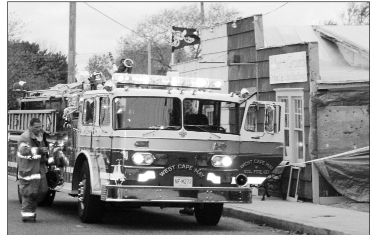
Above, fire crews from West Cape May and Cape May Point responded to a fire in a building that houses Key West Tacos and Higher Grounds Coffee Shop at Park and West Perry, Tuesday. Cape May Point Deputy Fire Chief Mike Mahon said there was significant damage, but it was not a total loss.
